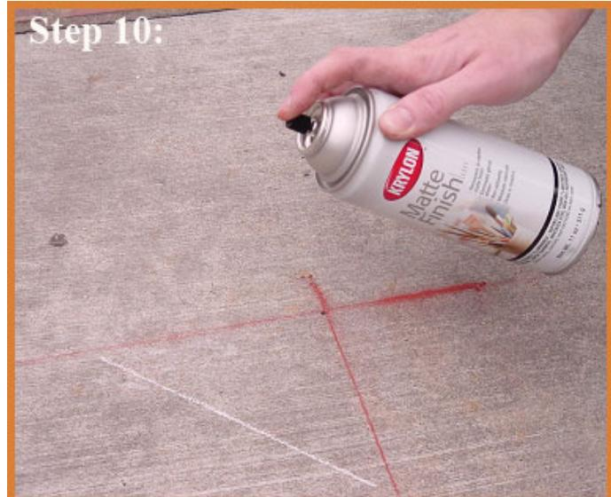
**Protect the chalk lines made by spraying a clear coat or matte spray over the lines. This will protect the pattern from water (often used with a saw-cut machine) and wind. To complete the installation follow the instructions supplied with the loop.**
