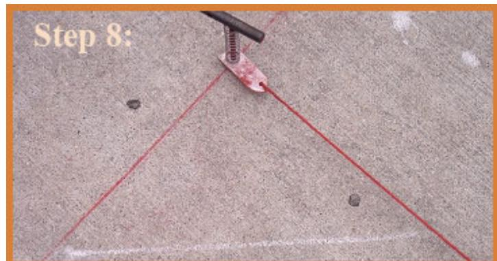
Remove "T" pins from the ground. Use the modified Chalk line to mark the loop pattern by inserting the chalk line's "T" pin into the holes drilled in the previous steps. Align the string over the corner hole and snap all four sides.
