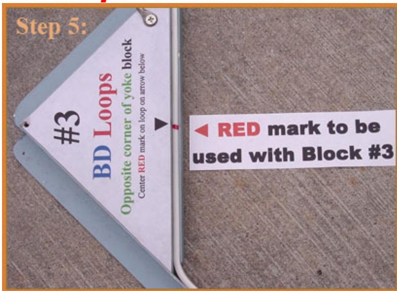
Ensure the loop wire has no twists, then find, align, and insert the red mark (already placed at the factory) into the arrow of block #3. Align block #3 with #2. Pull block #3 tight, drill a hole, then insert "T" bar to hold block #3 in place.
