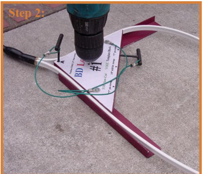
Position the #1 block where the loop yoke will be installed. Use the supplied 1/8 inch masonry drill bit to drill a hole (through previously drilled guide hole on the block) into the roadway surface. Drill a second hole to align the #1 block to form a 90° corner. Insert "T" bar into the holes.
