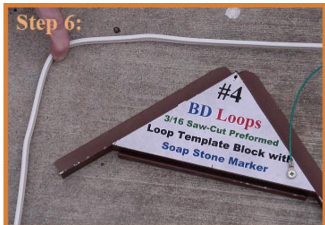
Pull the last corner of the loop with your finger to make a  $90^\circ$  angle and make a mark on the loop. Align and insert the mark into the arrow of block #4. Align so the wire is tight, drill a hole, and insert "T" bar to hold block #4 in place.
